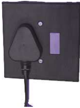
Fig.2. shows switching ON the power supply
